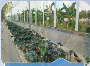
Station 12: Sewerage ditch connected to agricultural demonstration area of VRU.
